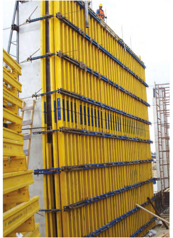
H20 wooden beams gives the opportunity of obtaining different heights connecting by H20-H20 band connecting element and using them as one beam.
