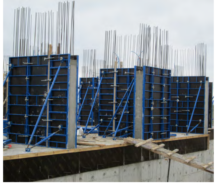
Thanks to its adjustable lite panels, different sizes of columns and It allows the manufacture of curtains.
